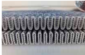
The Filter Media has absorbed water
